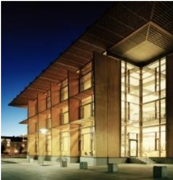
Figure 22. Photographs of the Mälardalen University library built with wood-frame and glass in Västerås. (Photograph credit: Åke E:son Lindman).
